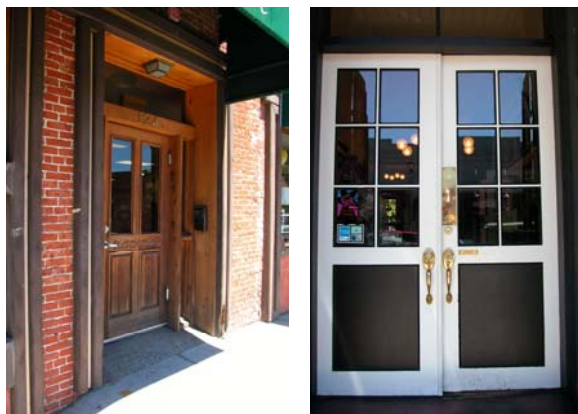
Examples of new doors that reflect the design and materials of the originals.
