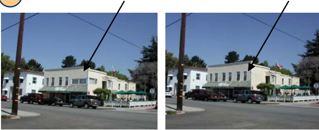
Example of an inappropriate modification (left) to the original (right) window configuration.
